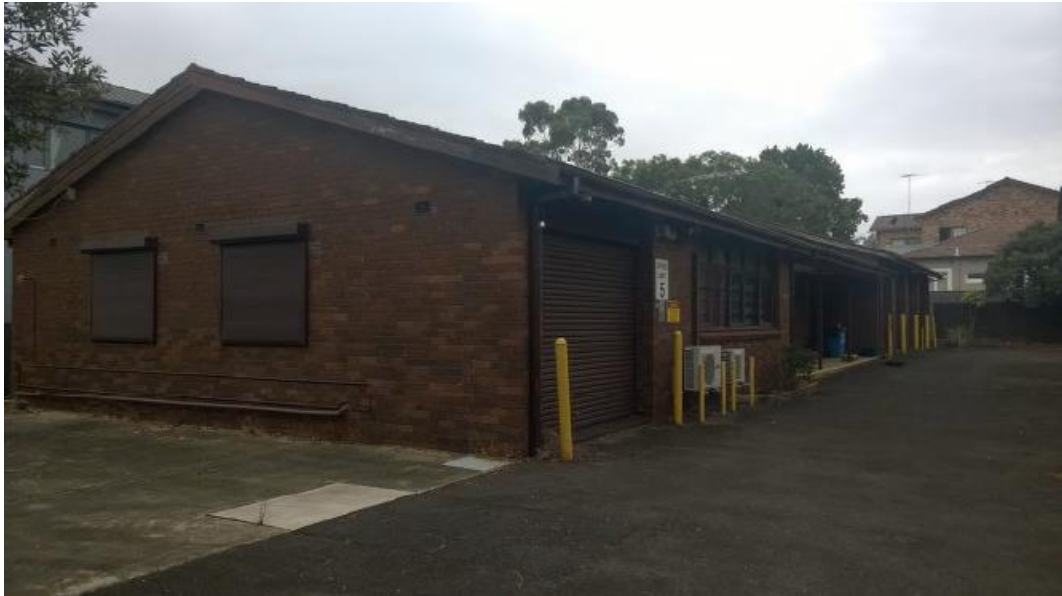
Figure 29: Depot Building (Lot 95 DP 6743) – to be demolished
