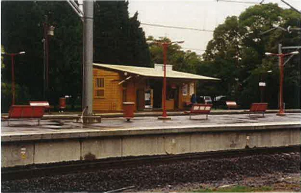
Figure 18: Concord West Railway Station-1998
