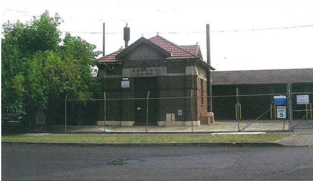
Figure 28: MWS & DB Pumping Station – 32 Wymston Parade 2007
